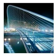
His name, Zubizuri, means White Bridge in Euskera but is also known as Calatrava's Bridge. This footbridge consists in a slim arch that supports the bridge deck built in transparent and translucent glass bricks. It seems that you are walking on the air over the Nervion River! It is located very near the Guggenheim Museum.
